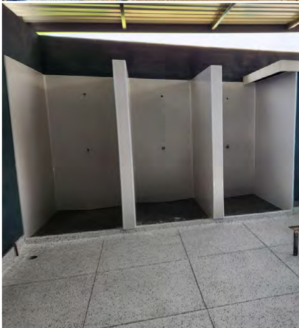
Photo: Swimming Change Rooms Restoration
