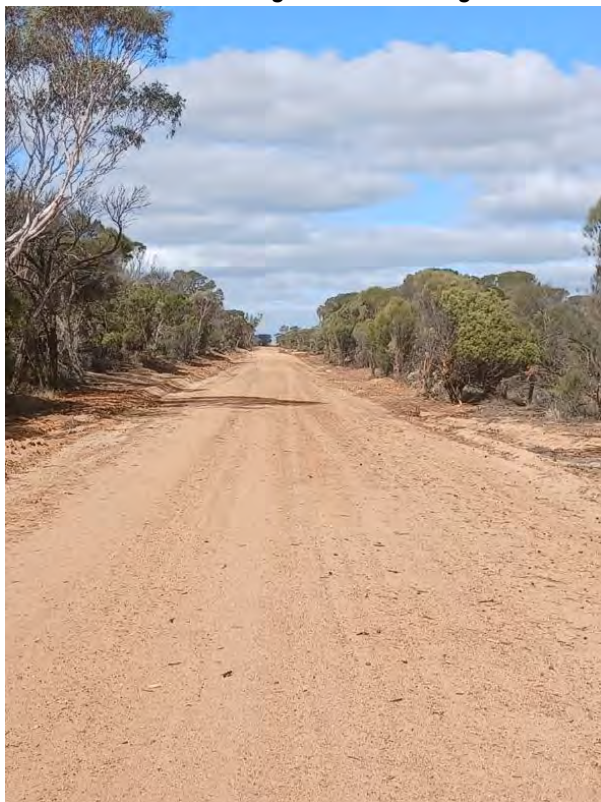
Photo: Gangell Rd – Vegetation Clearing
