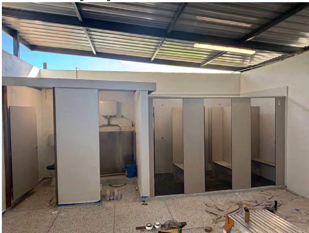
Photo: After Pictures - Swimming Change Rooms Restoration
