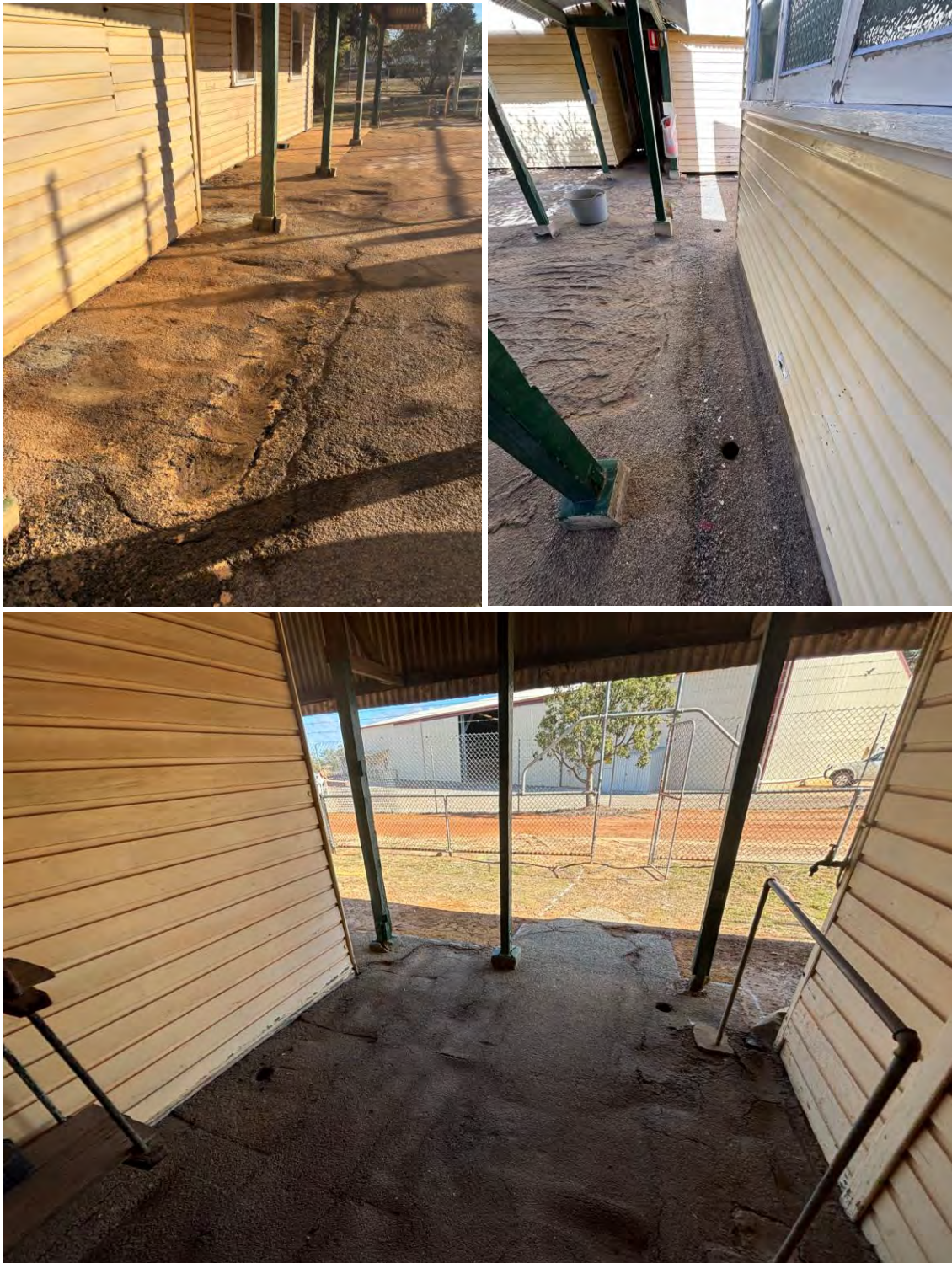
Photo: Before Pictures - Railway Barracks Accommodation
