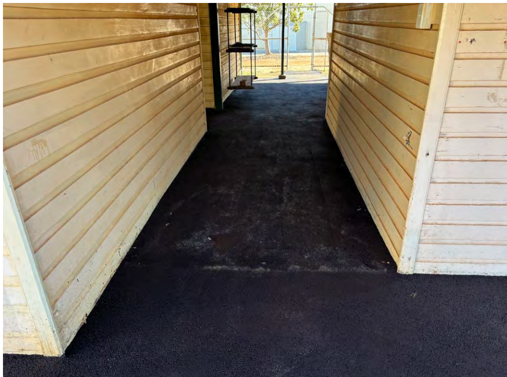
Photo: Before Pictures - Railway Barracks Accommodation
