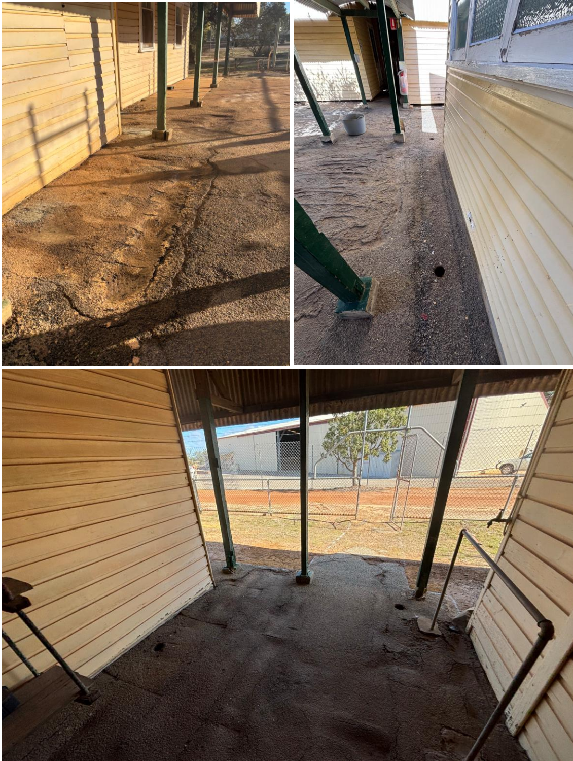
Photo: Before Pictures - Railway Barracks Accommodation
