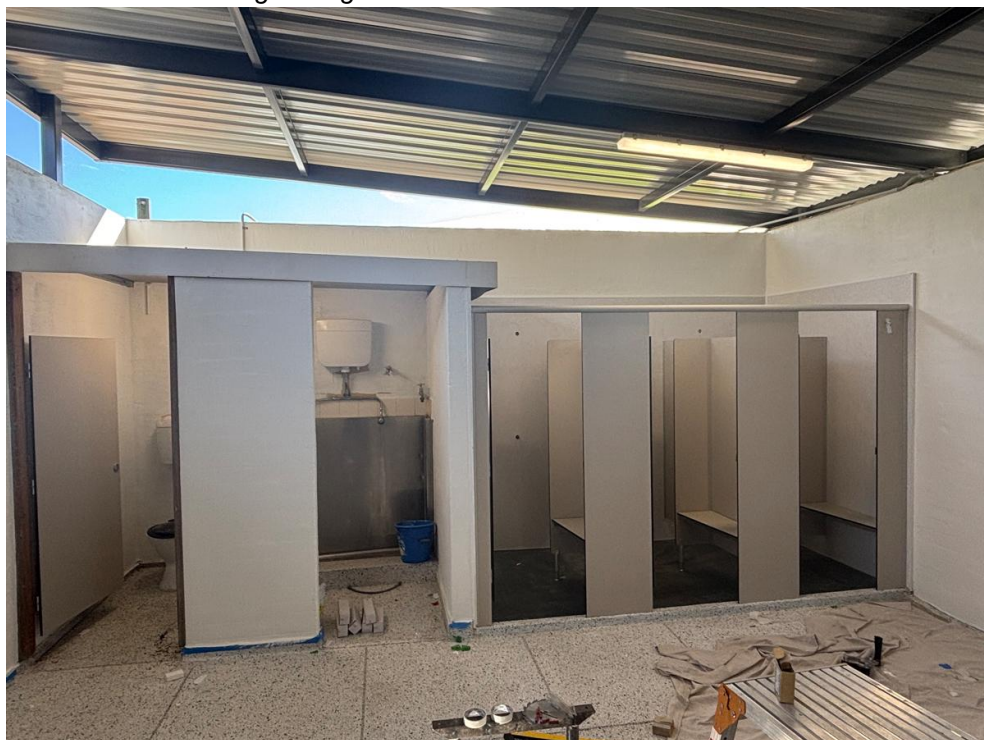
Photo: After Pictures - Swimming Change Rooms Restoration
