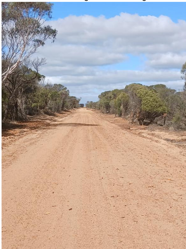
Photo: Gangell Rd – Vegetation Clearing
