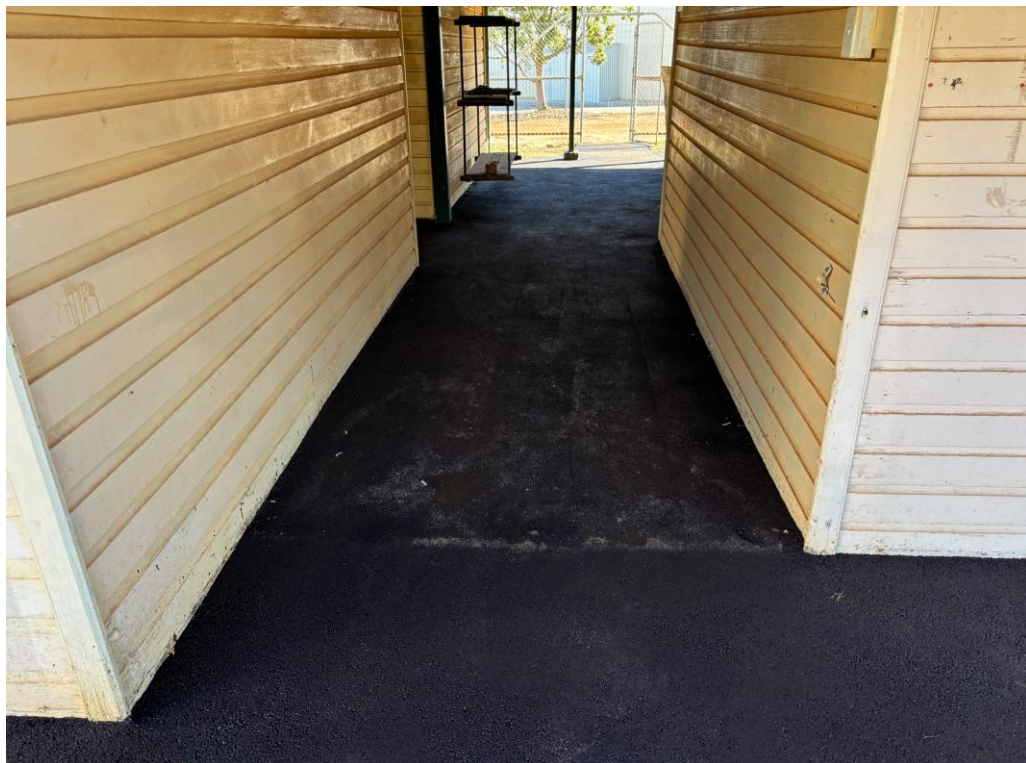
Photo: Before Pictures - Railway Barracks Accommodation
