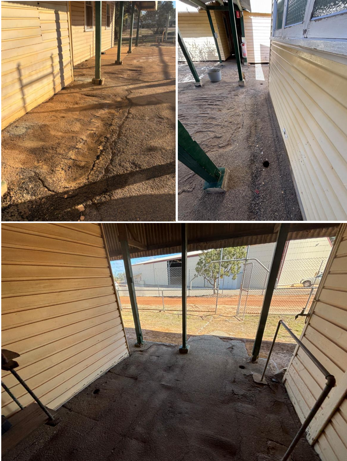
Photo: Before Pictures - Railway Barracks Accommodation
