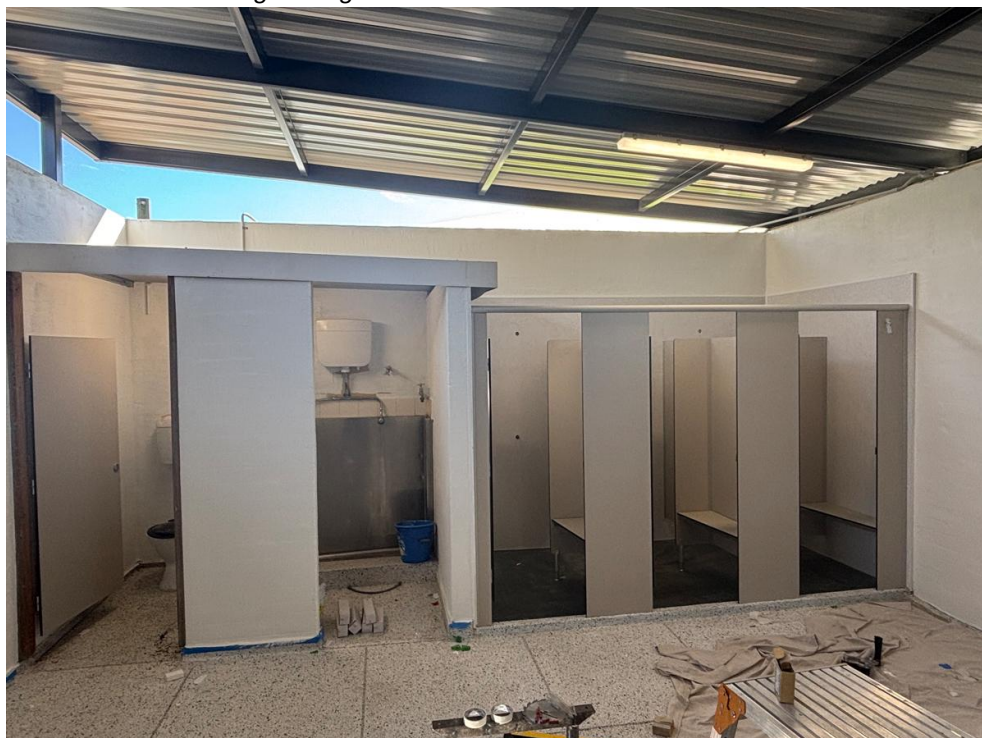
Photo: After Pictures - Swimming Change Rooms Restoration
