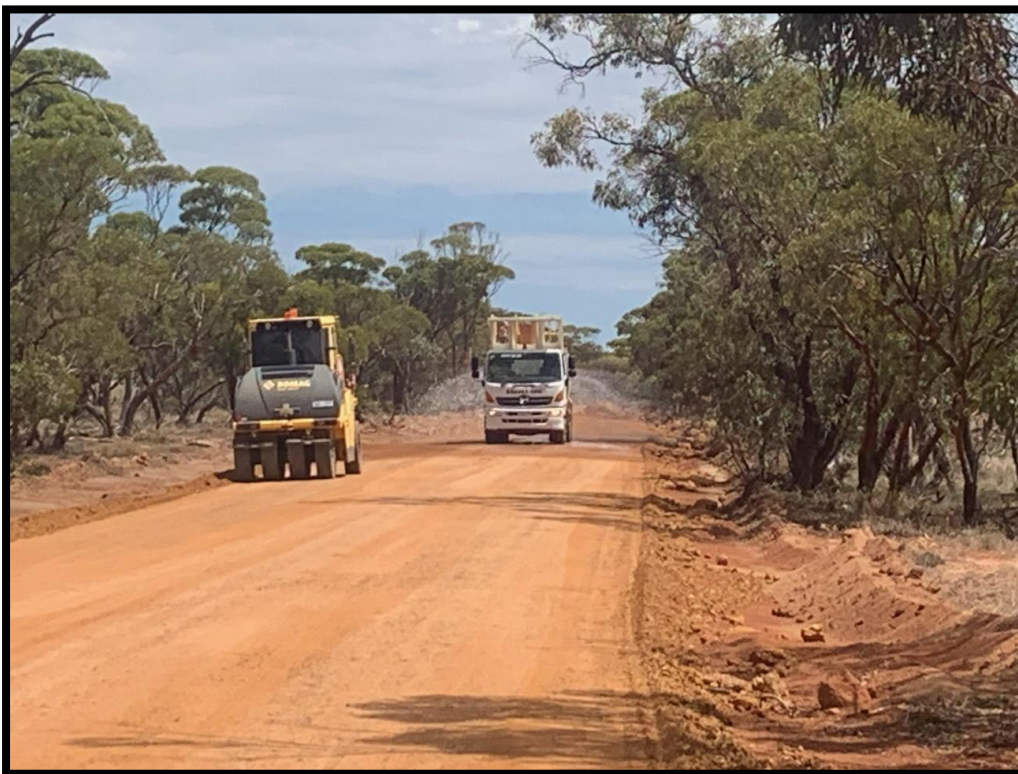
Capital works Minnivale North East Road.
