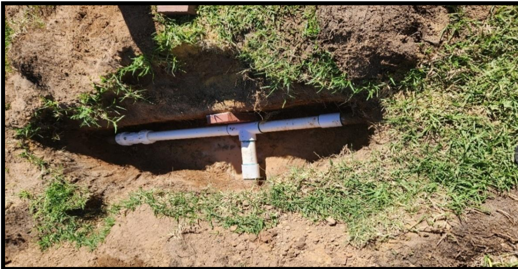
Burst mains pipe under the lawn at the swimming pool.
