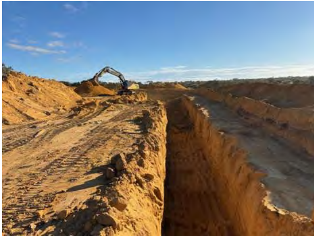
Photo: Refuse Site – New Cell Excavation
