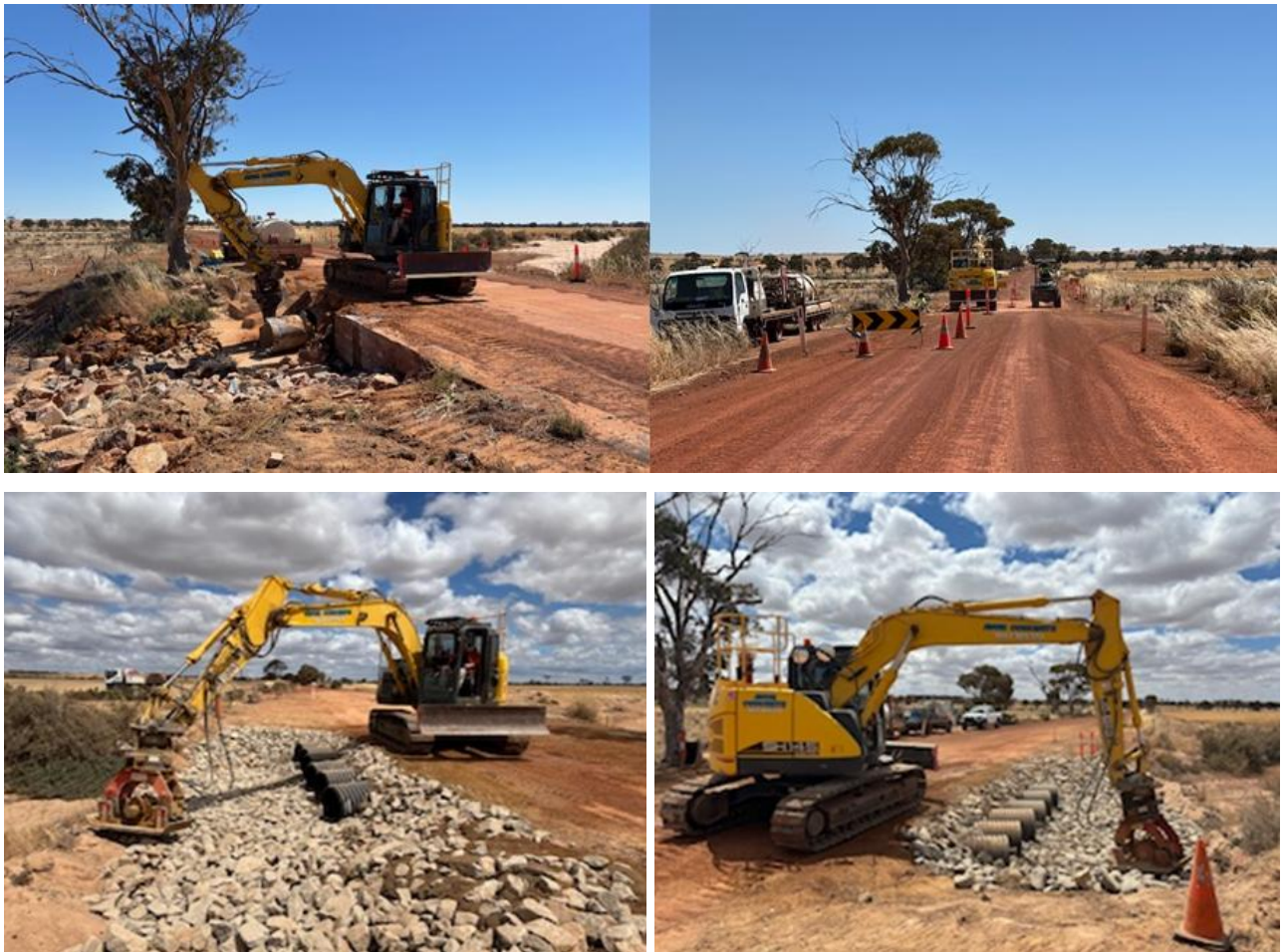
Photo: Davies Rd SLK 20.47 - Culvert Replacement (Roads to Recovery)
