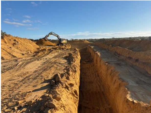
Photo: Refuse Site – New Cell Excavation
