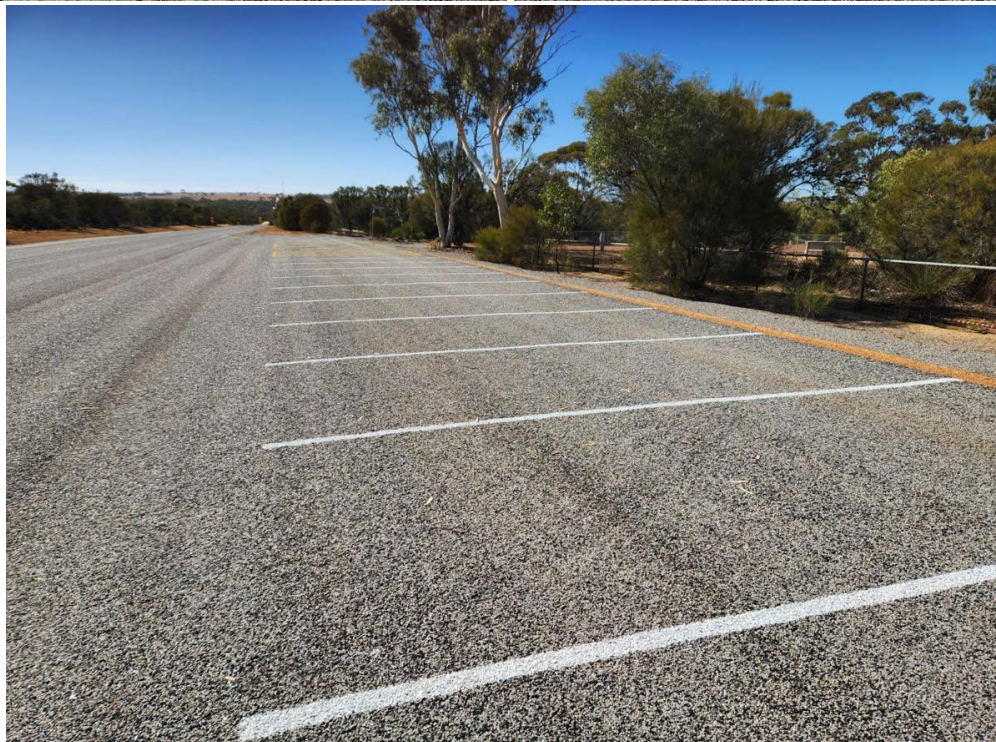
Photo: Cemetery – Car Park Line Marking
