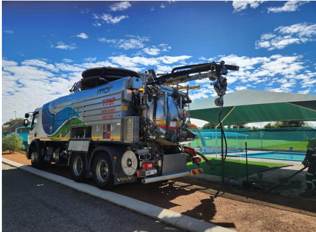
Photo: Swimming Pool – Septic Tank cleaning and jetting.
