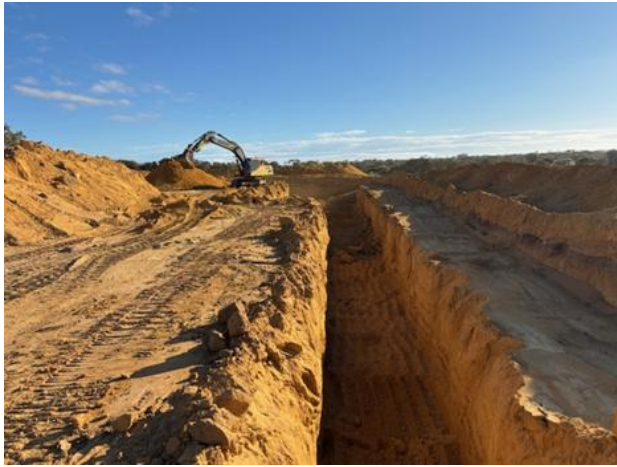
Photo: Refuse Site – New Cell Excavation
