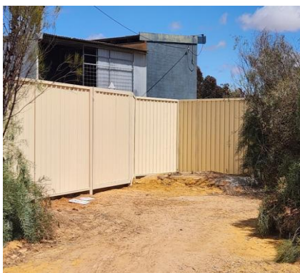
Photo: Swimming Pool Pump Station
