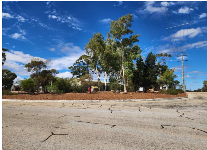
Photo: Mulching Works within the Town site.
