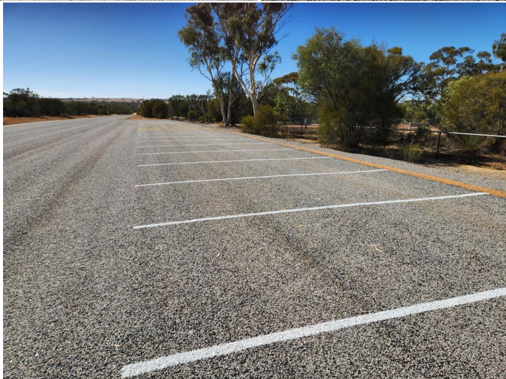
Photo: Cemetery – Car Park Line Marking
