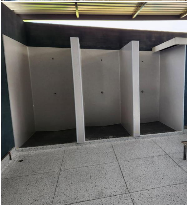
Photo: Swimming Change Rooms Restoration
