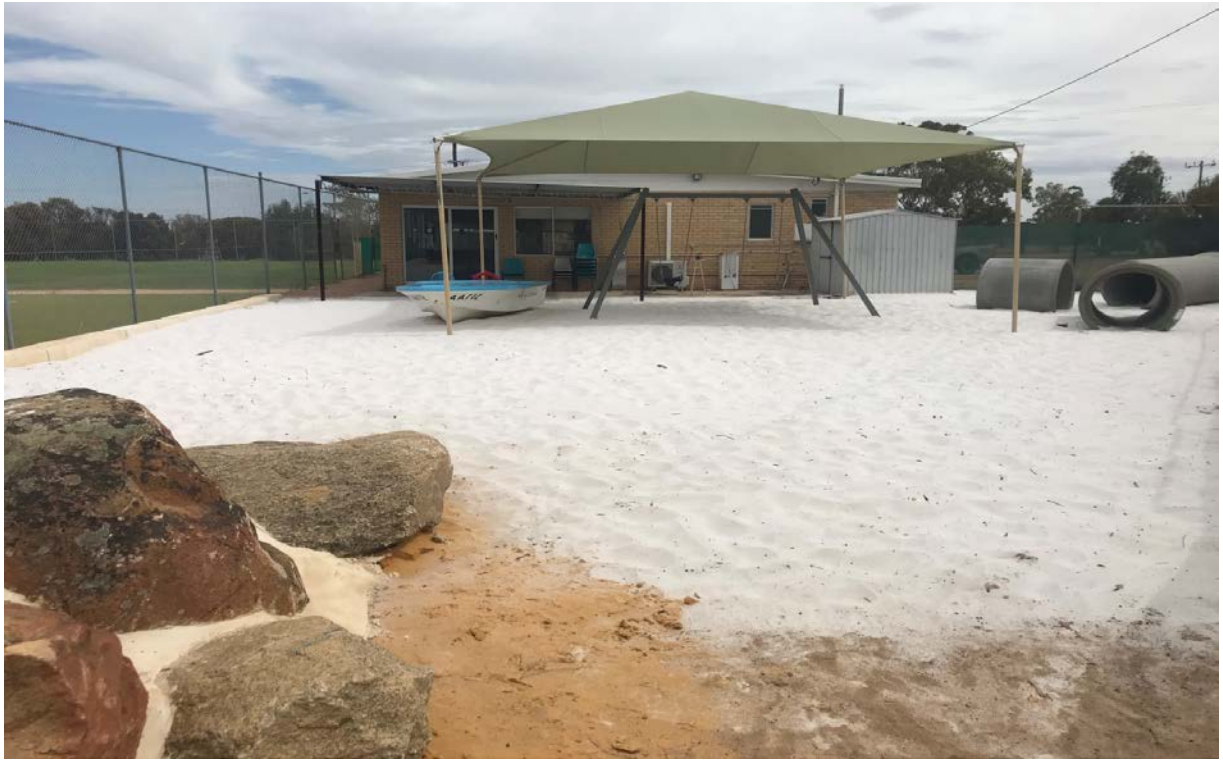
Playground all finished looking west.
