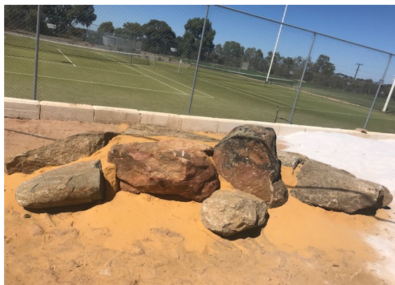
Climbing Rocks in place ready to be cemented in
