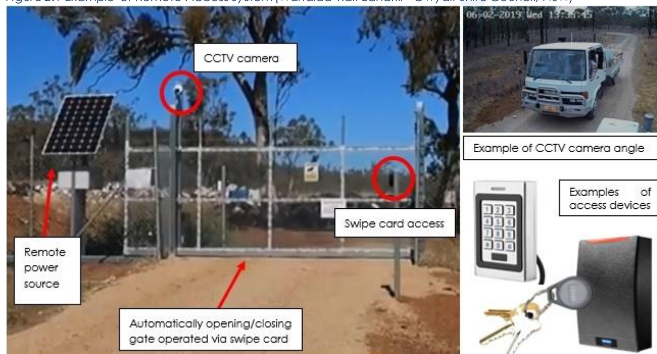
Figure 2.1 Example of Remote Access System (Warialda Rail Landfill - Gwydir Shire Council, NSW)
