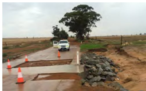
FLOODWAYS DAMAGED
